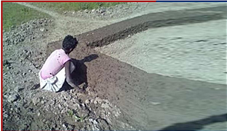
Household Beneficiary Constructs Plinth of His House Under ORS Project
