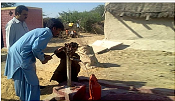
Hand Pump Installed for Drinking Water
